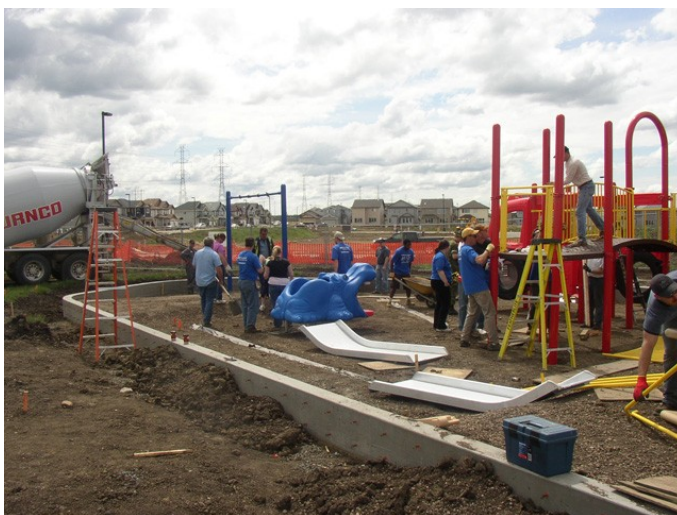
Construction Of The Silverberry Playground In The Meadows Community League
