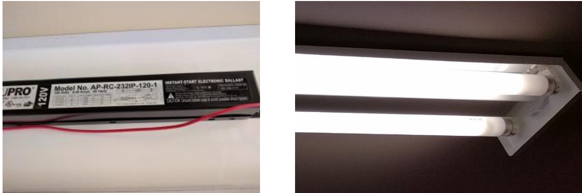
FIGURE 9. T8 INSTANT-START ELECTRONIC BALLAST (LEFT) AND T8 FLUORESCENT LAMPS (RIGHT)
