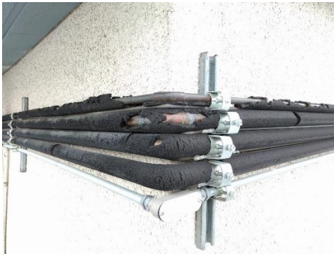
FIGURE 26. DEGRADED FOAM INSULATION ON AIR CONDITIONER REFRIGERANT LINES (LEFT) AND UV-RESISTANT PVC JACKETING FOR PIPE INSULATION (RIGHT)
