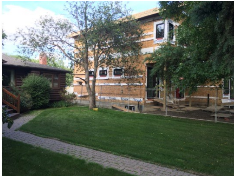
Image 4: Photo of a development in Windsor Park, Edmonton that dwarfs its neighbour due to changes to front set back regulations.
